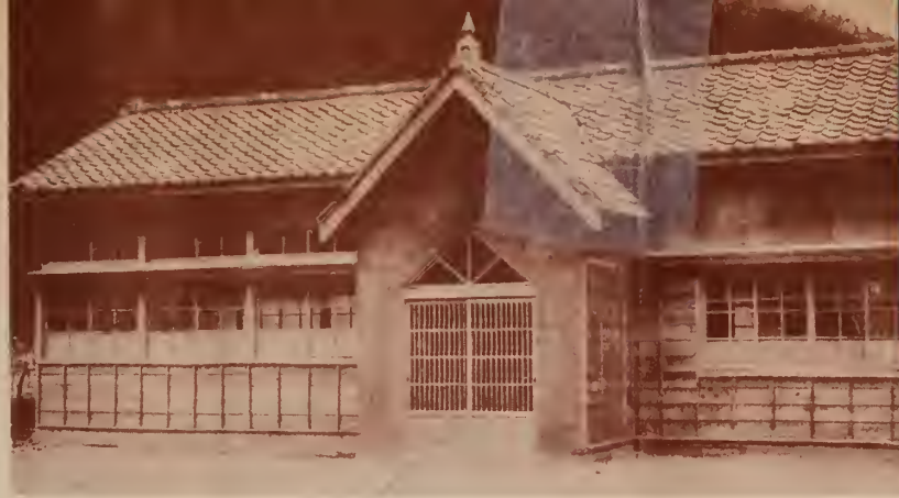
New Kindergarten building at Nakazuma, Japan. Dedicated June 1, 1941. Page 309.
